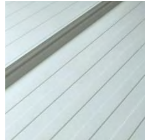
STANDING SEAM ROOF
